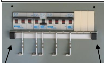
Lower/Raise Rod by turning Brackets around. Holes close to slots must be used.
